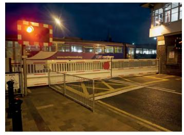
The first train passes newly installed sliding-gate level-crossing barriers at West Dyke Road, Redcar in December 2015. Developed and supplied for Network Rail by EDS Ltd, they incorporate position/rotation sensors and a programmable logic controller to vary speed dependant on the position of the gate, and have 'fast stop' edge sensors. The previous boom gate barrier was plagued by reliability problems during high winds. Network Rail
