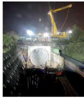
The new tunnel at Farnworth near Bolton opened to passenger services on 14 December 2015. One of the two existing tunnels was enlarged to accommodate two tracks and overhead electrification. Network Rail
